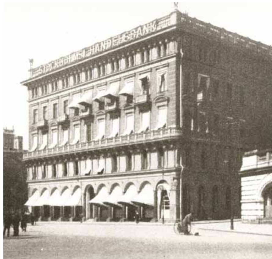
Since spring 1905, Handelsbanken's head office has been situated at Kungsträdgårdsgatan in Stockholm.
