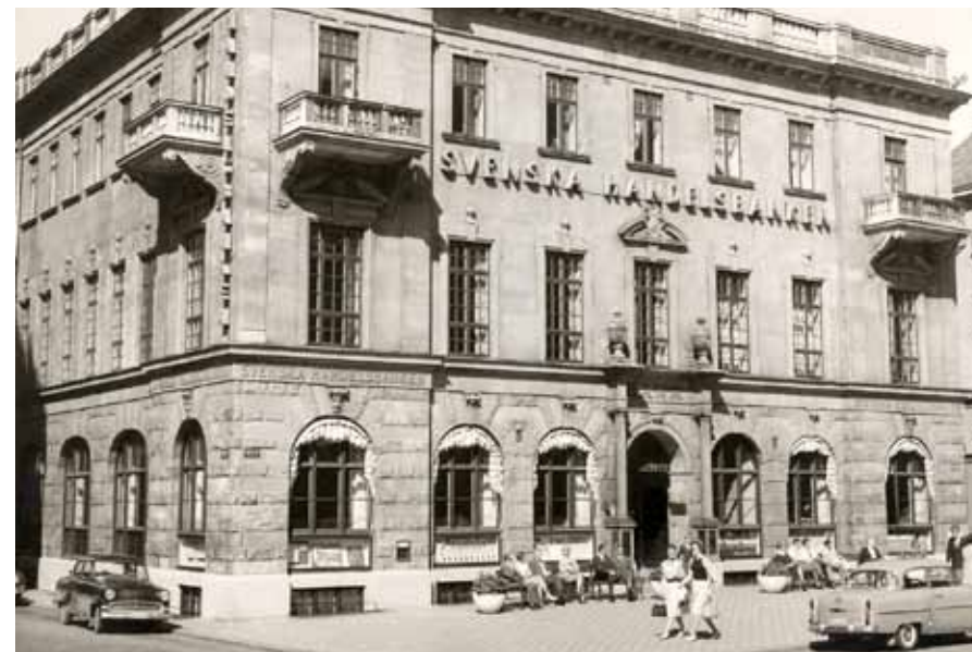
Handelsbanken's branch at Stortorget in Helsingborg in the 1950s. Handelsbanken took over the building, which was previously the headquarters of Bankaktiebolaget Södra Sverige, in 1919.
